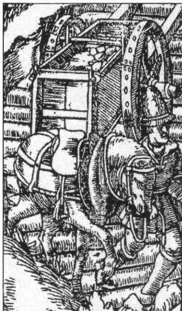
Fig.18 Illustration from 'De Re Metallica' of a narrow cart used in Iron mining.
